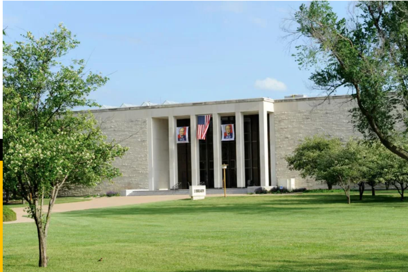
Eisenhower Library Source: Architectural Digest
