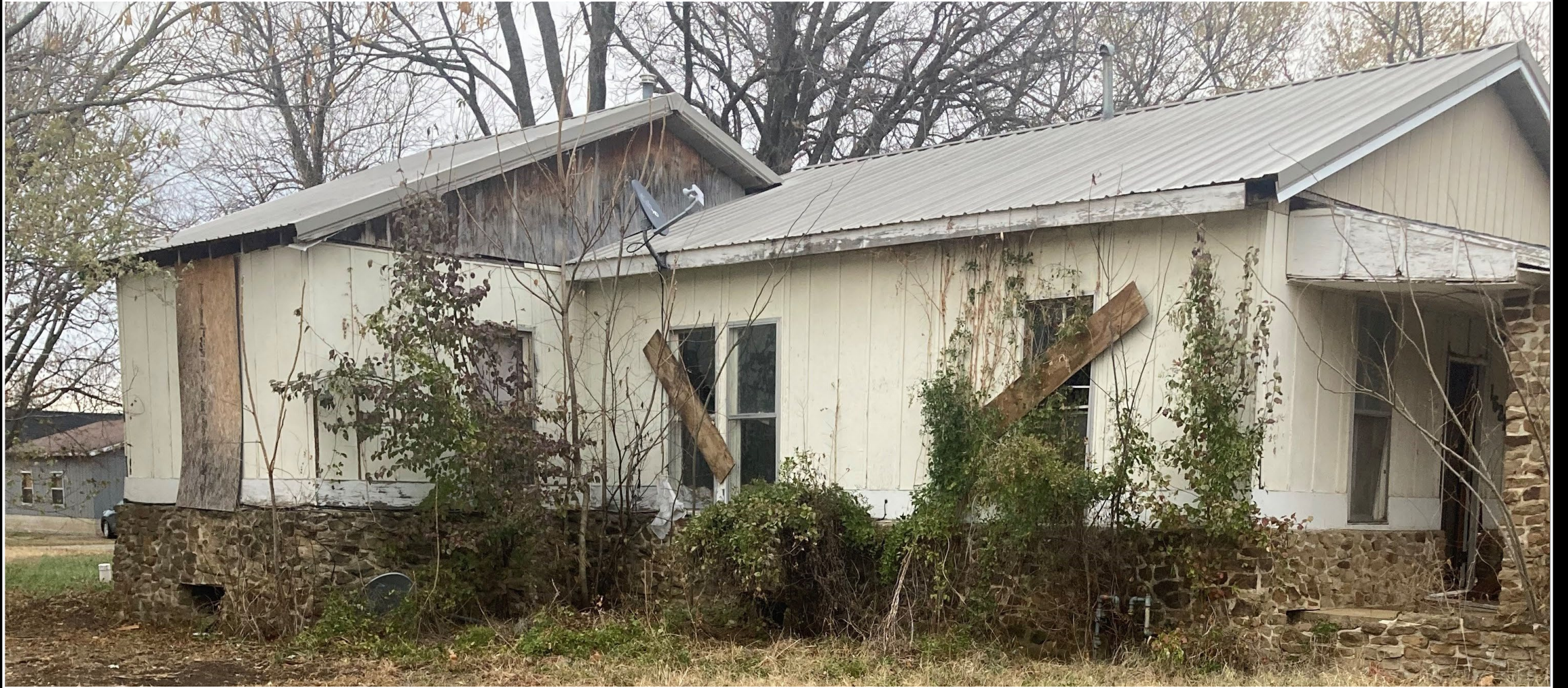
Infill – Demolition * Land Bank 1621 Chess
